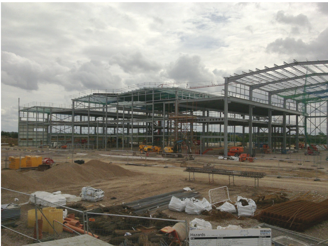
The Manufacturing Technology Centre under construction 20th August 2010
